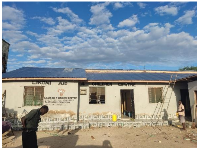
Newly replaced roof with improved protection
