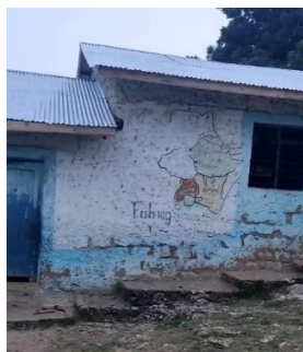
Newly replaced roof with improved protection
